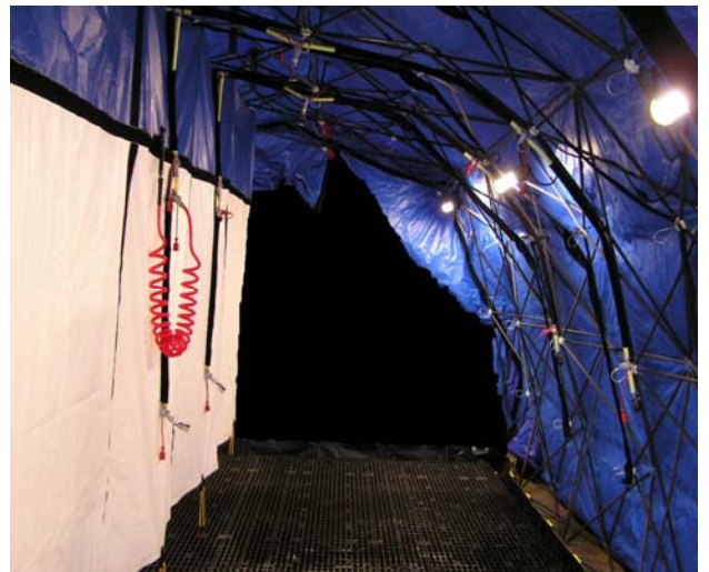
Figure 2-10. Internal Plumbing
