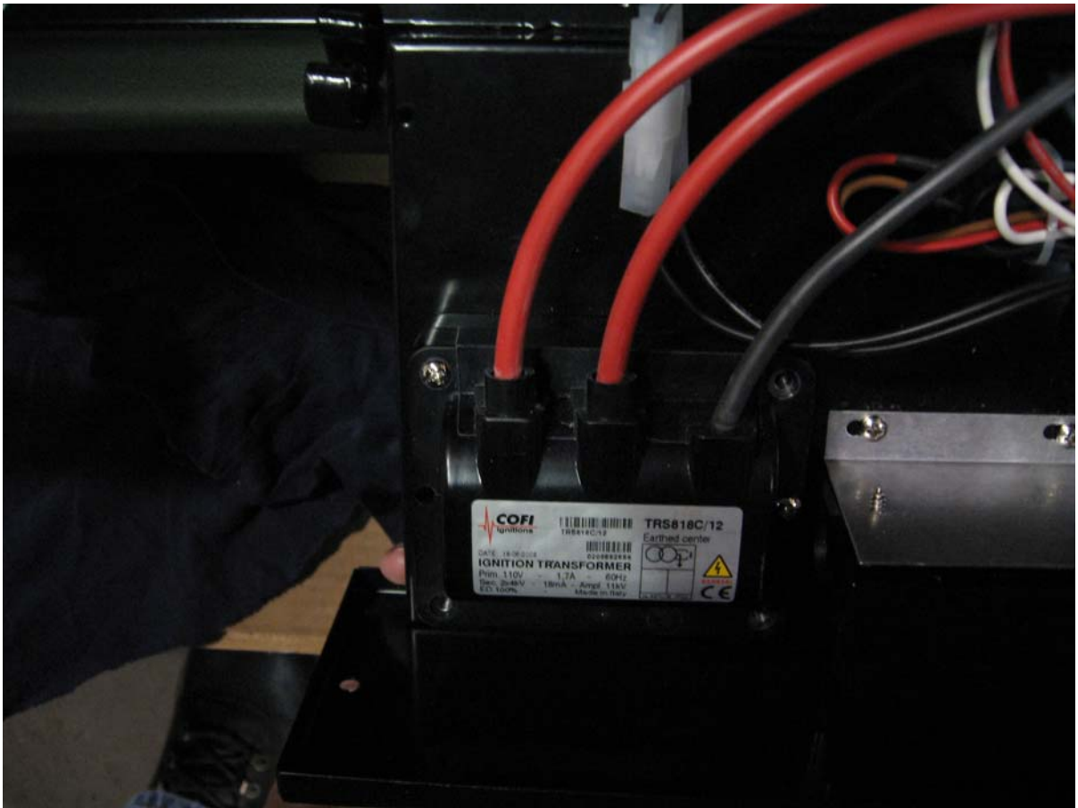
Figure 5-11 - Transformer and H.T. Leads
