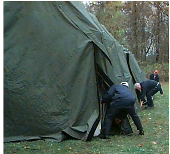
Figure 3-28 - Pulling Out the Wall
