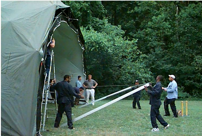
Figure 3-18 - Lifting the end wall into place
