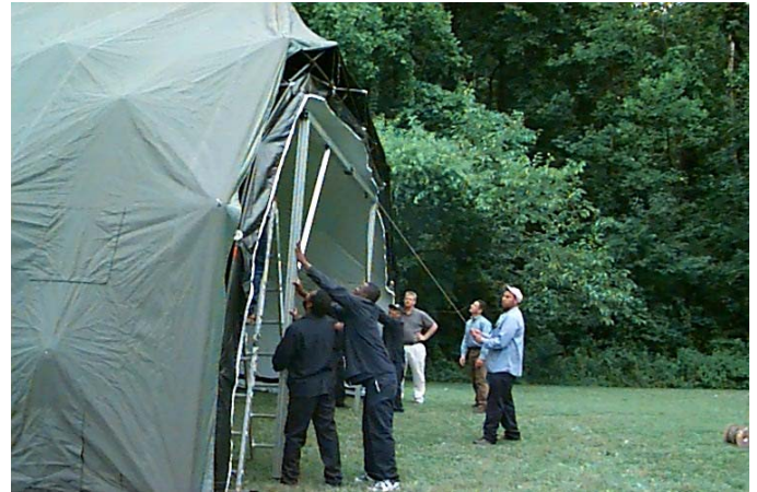
Figure 3-19 - Securing the end wall into place
