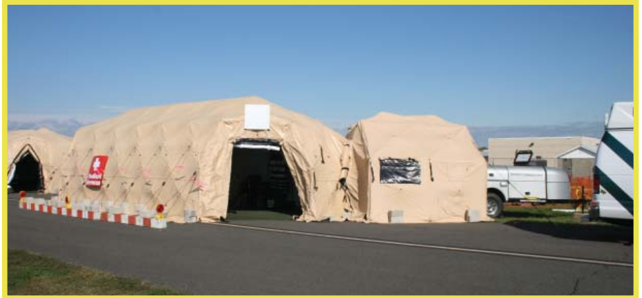
A DRASH 6XB is booted at a Reeves Incident Command Post (ICP), completing the medical shelter set up during an air show at Brainard Airport.
